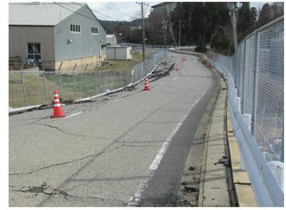
(c) 壁体背面地盤の沈下
